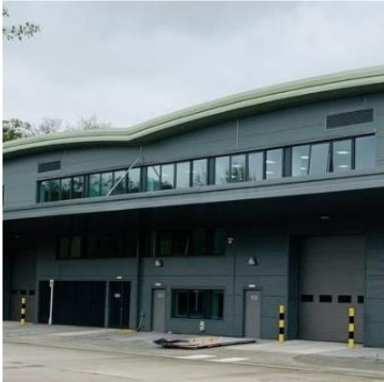
Building upgrades or new buildings ISO 14001 certified production sites: covering around half of sales Bucher Municipal's new hall in Dorking
