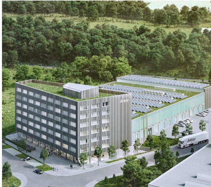
Bucher Automation, Marbach, Germany
